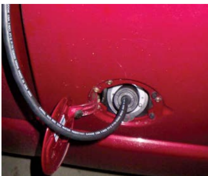
The AC input for the battery charger is accessed through the old fuel filler door.
